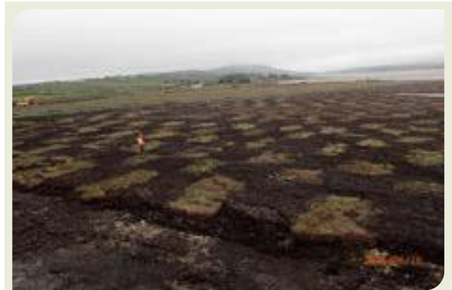
Plate 16a: Aughooose - overview of matrix of vegetated blanket bog turves and bare peat during the reinstatement of the former tunnelling site compound
