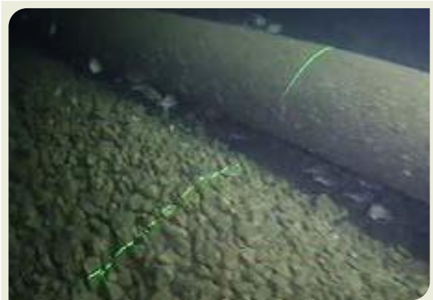
Plate 7b: Rock span protection water depth 80m
