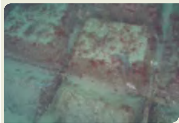
Plate 5a: Concrete Mattresses
