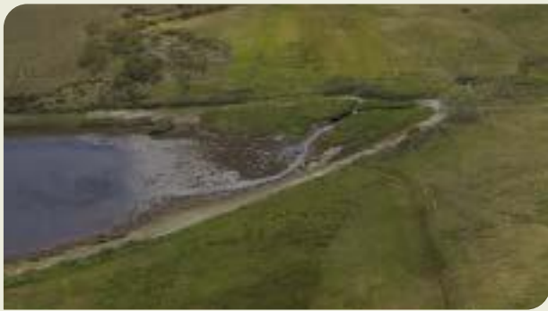
Plate 21b: Aerial of Leenamore inlet, two years after construction and salt marsh reinstatement
