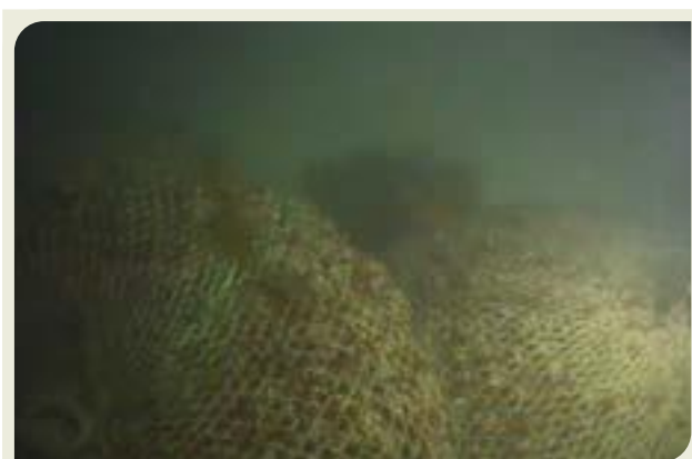
Plate 5c: Mesh rock bag protection (filter units) Water depth 25m
