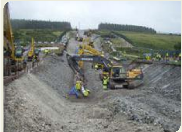
Plate 24: For comparison with Plate 23, pipelaying at the Leenamore inlet in 2013 (facing east across the inlet)
