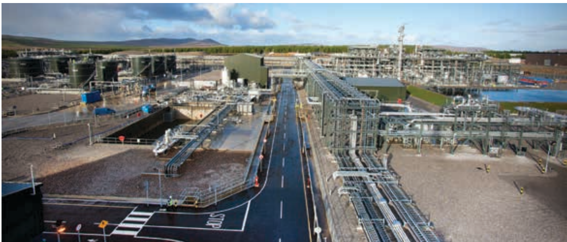
Bellanaboy Bridge Gas Terminal nearing completion
